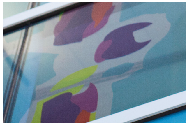
Detail of curtain wall above. ViviGraphix Spectra glass in View configuration with Custom graphic interlayer
