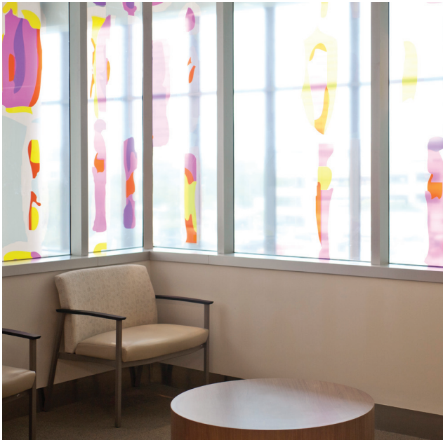
Curtain wall as seen from Operating Room waiting area
