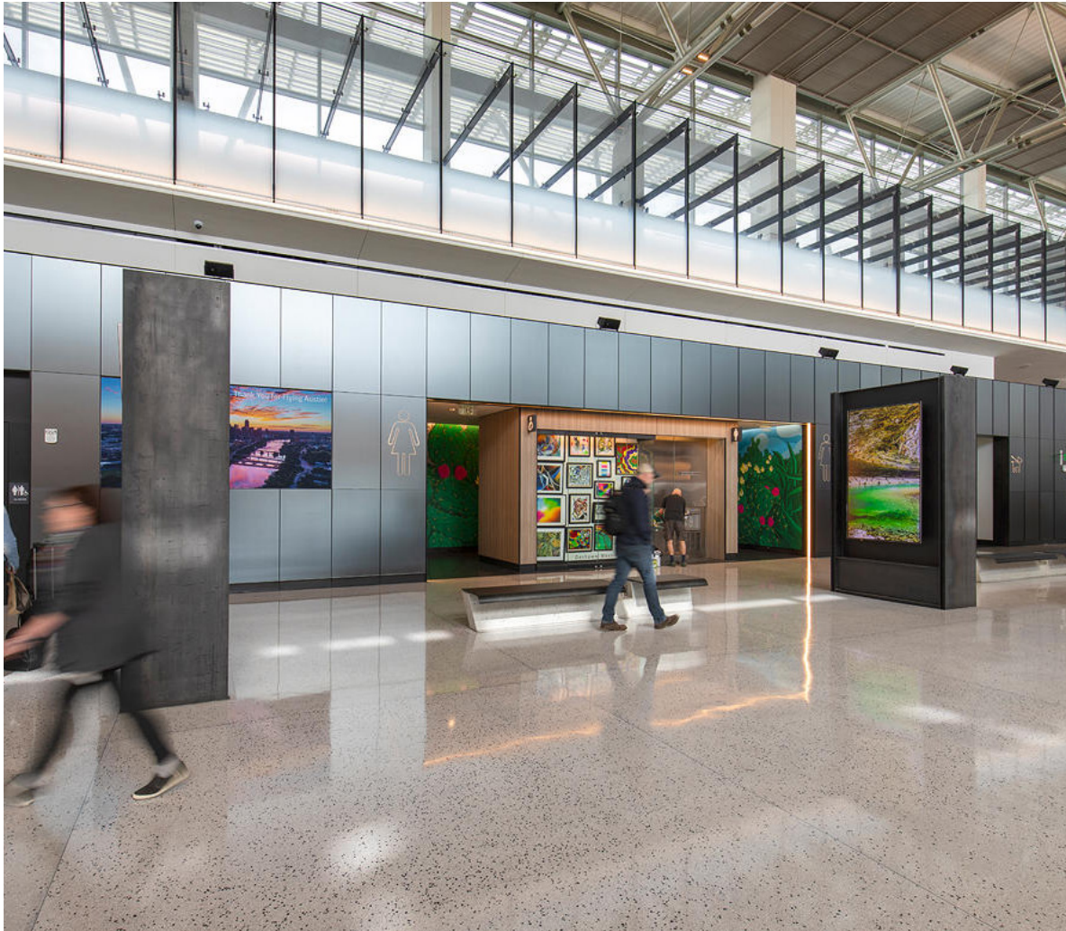
Austin-Bergstrom International Airport, Austin, Texas | Left, Top & Opposite LEVELr Wall Cladding System with panels in ViviChrome Chromis glass with custom color interlayer and Opalex finish, and custom reveal fins in black; upper-level corridor with ViviGraphix Gradiance glass with Vapor pattern interlayer and Standard finish
