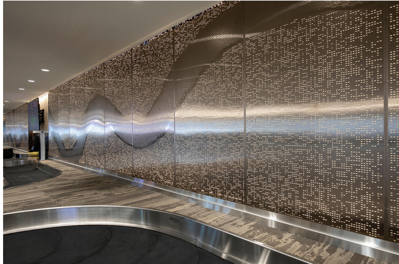
Louis Armstrong New Orleans International Airport, New Orleans, Louisiana | Opposite Feature wall with ViviSpectra Spectrum glass with custom image interlayer and Pearlex+ finish
