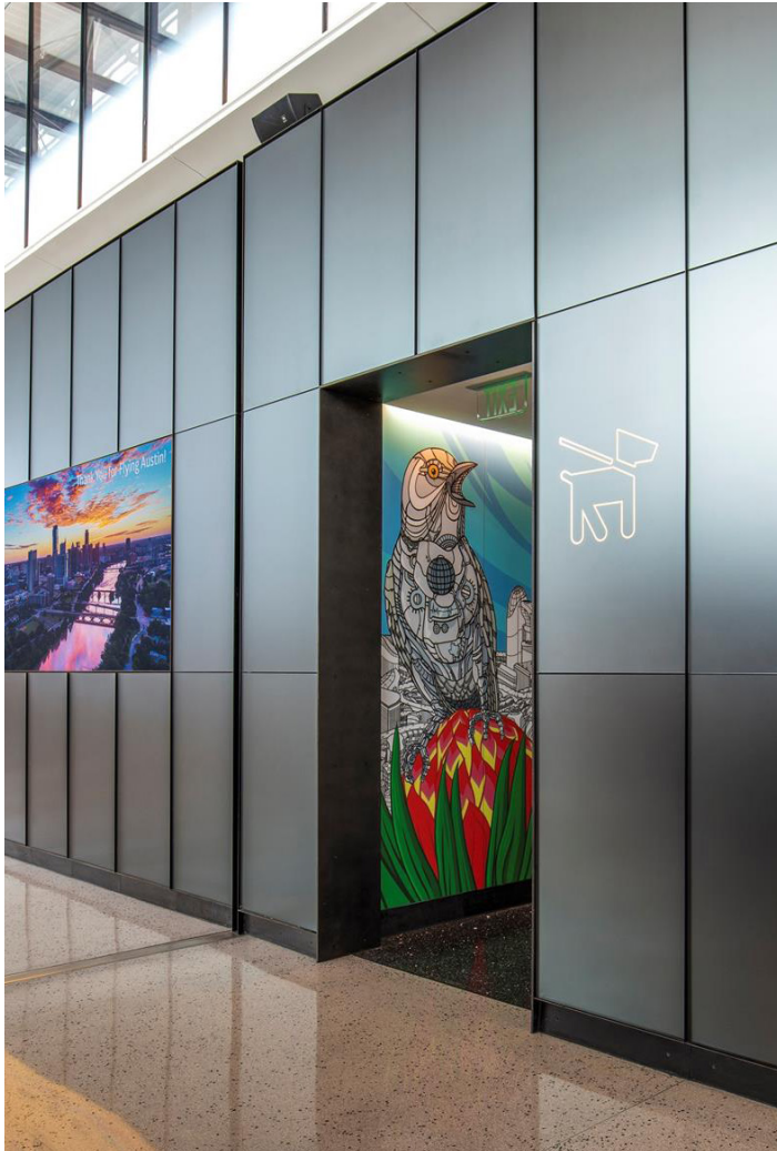
Austin-Bergstrom International Airport, Austin, Texas | Left Custom restroom graphic with custom LightPlane backlighting in LEVELr Wall Cladding System with panels in ViviChrome Chromis glass with custom color interlayer and Opalex finish
