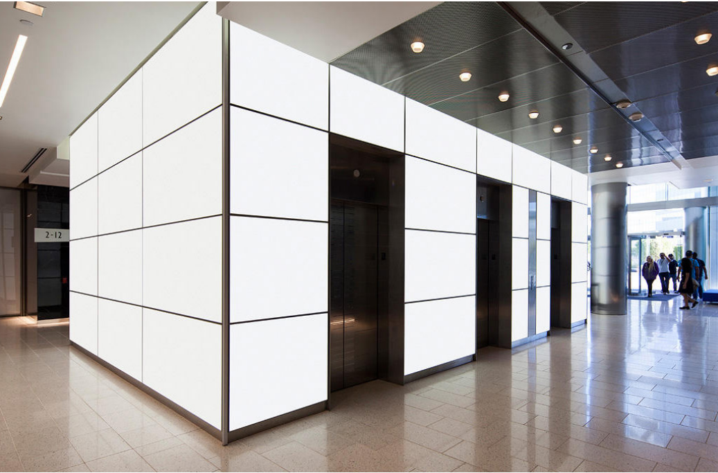
Pacific Corporate Towers, El Segundo, California | Top & Right LEVELe Wall Cladding System with LightPlane Panels in ViviChrome Chromis glass with White interlayer and Opalex finish
