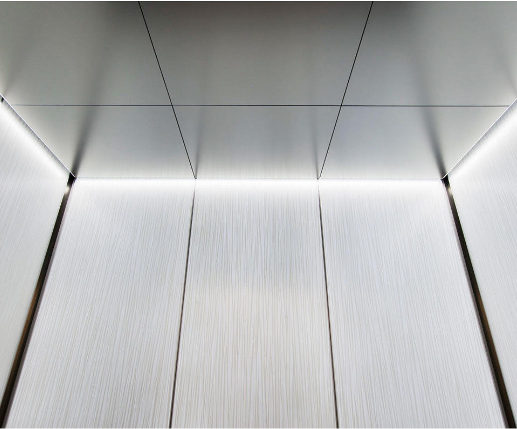
Private Location, New York, New York | Left Elevator Ceiling in Stainless Steel with Seastone finish; LED perimeter lighting
