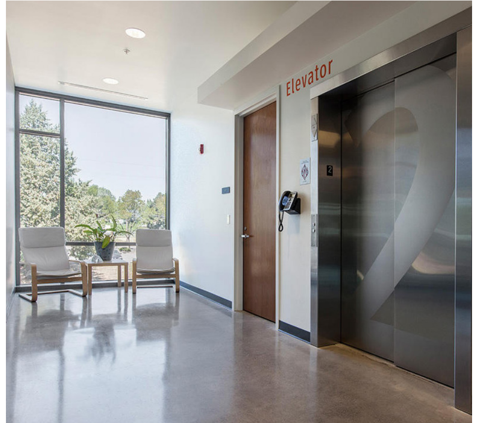
Herb Chambers, Boston, Massachusetts | Top Elevator Doors in Bonded Nickel Silver with Dark Patina and Vancouver pattern
