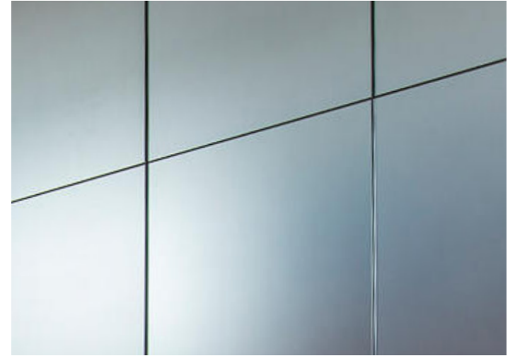
Austin-Bergstrom International Airport, Austin, Texas | Left, Top & Opposite LEVELr Wall Cladding System with panels in ViviChrome Chromis glass with custom color interlayer and Opalex finish, and custom reveal fins in black; upper-level corridor with ViviGraphix Gradiance glass with Vapor pattern interlayer and Standard finish
