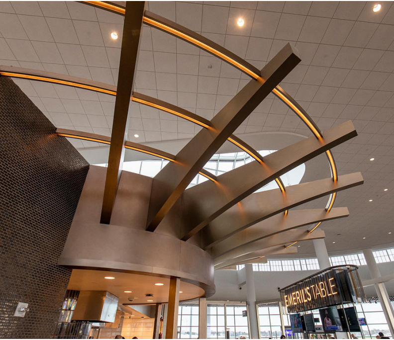
Louis Armstrong New Orleans International Airport, New Orleans, Louisiana | Left Architectural spokes and curved wall in Fused White Gold with Seastone finish
